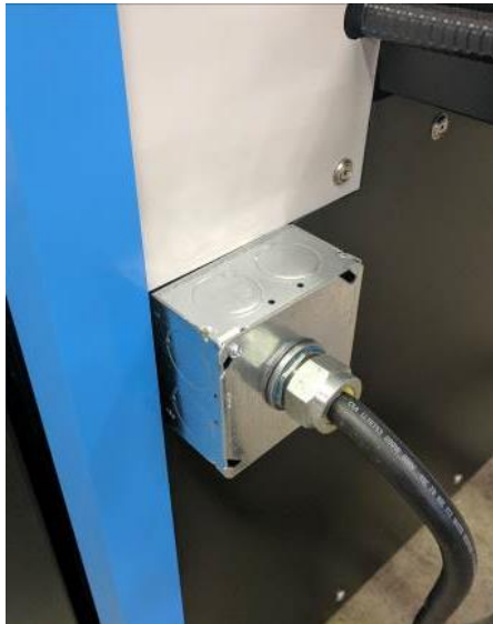
Figure 4. Power Supply Wiring
