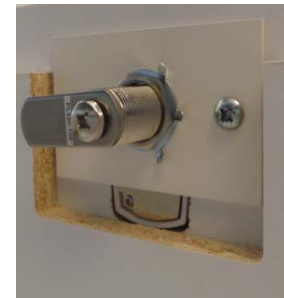
Photo indicates Arm position for unlocked Cam Lock
