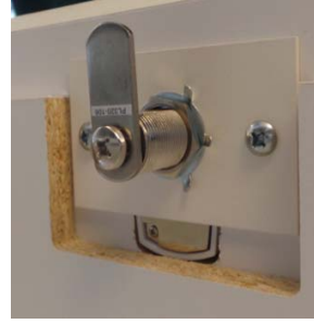
Photo indicates Arm position for locked Cam Lock.
