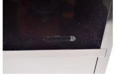
Use a router tool to route the pocket to a minimum depth of 12.7mm (0.5 in). Drill the screw holes using a 2mm (0.08 in) drill bit.
