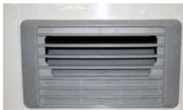
2. Pull the filter grate from the bottom up until it unlocks from the wall.
