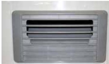
2. Pull the filter grate from the bottom up until it unlocks from the wall.
