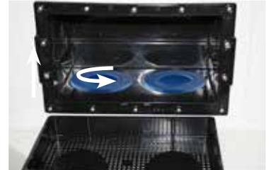
6. Pull filter up, then angle the top away from the filter compartment to pull filter completely out. Each filter has 4.5 m<sup>2</sup> of effective filter area.
