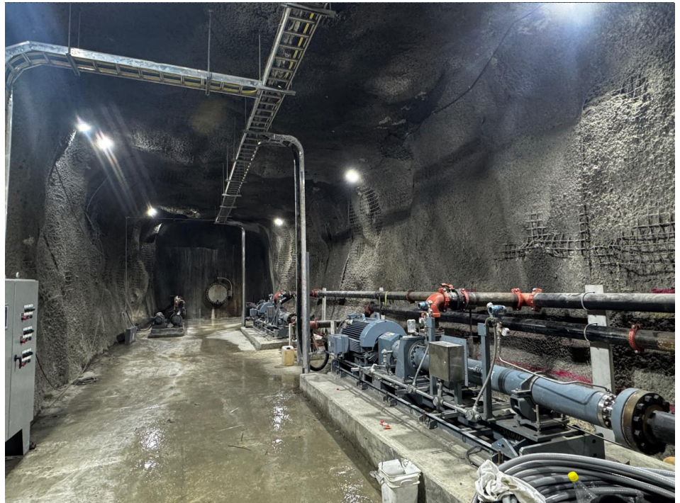
Two Hercules HPS SM18500 installed in a mine, each unit 8 stages, 250 hp, 520gpm at 570 psi
