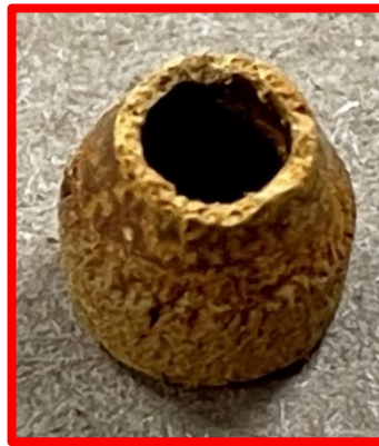
Leaking Ferrule – pitted and chipped surfaces (cleaned with harsh chemicals)
