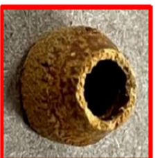
Leaking Ferrule: pitted and chipped surfaces (cleaned with harsh chemicals)
