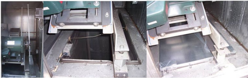
Use of sheet metal at supply air discharge from rooftop packaged unit to block off sealant from the coils and fans.
