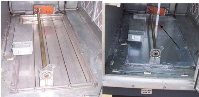
Use of sheet metal at supply air discharge from rooftop packaged unit to block off sealant from the coils and fans.
