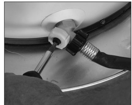
Figure 12 - Draining the old water heater.
