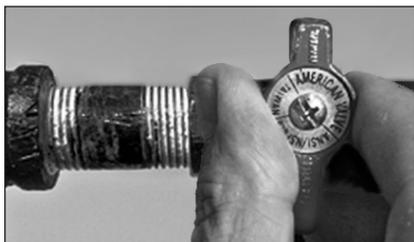
Figure 37 - Manual Gas Valve in OFF position.
