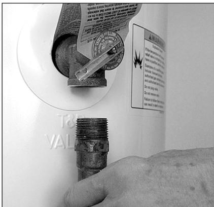
Figure 13 - Removing the T&P Relief Valve discharge pipe.
