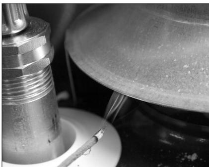
Figure 26 - Test the air supply and vent to make sure the water heater has adequate air and is venting properly.
