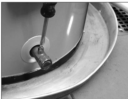
Figure 31 - Draining the water heater.
