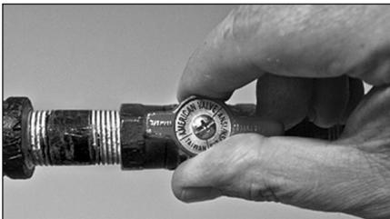
Figure 23 - Manual Gas Valve in ON position.
