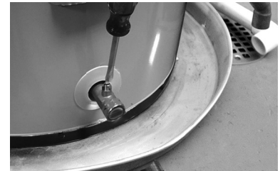
Figure 19. Draining the old water heater.
