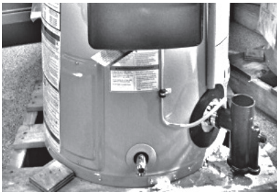
Figure 26. Condensate/Exhaust Tee Installation
