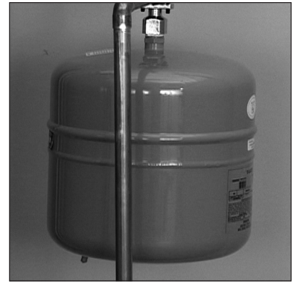
Figure 55. The Thermal Expansion Tank should be pressurized with air to match the home's incoming water pressure.
