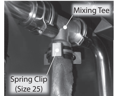
Figure 251 - Spring Clip (Size 25), Mixing Tee (B1)
