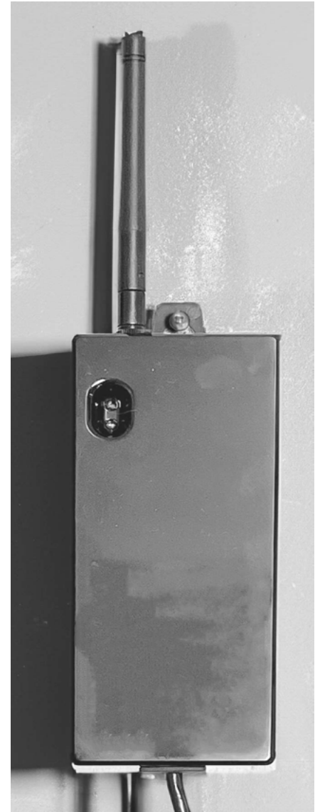
Figure 7 - Securing the remote recirculation receiver module to the wall
