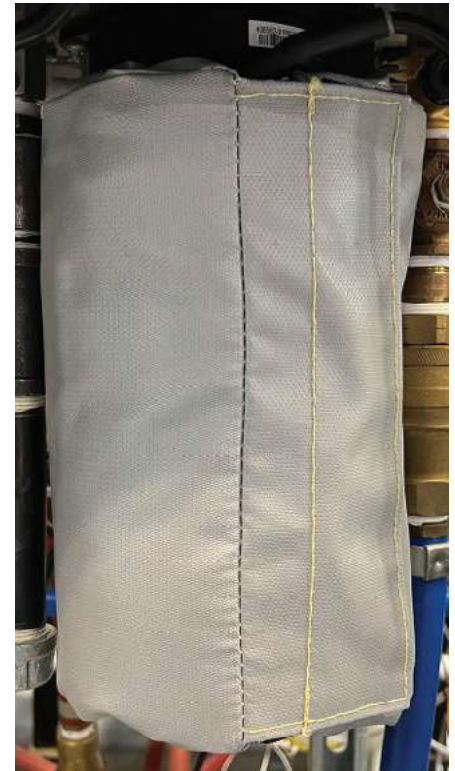
Figure 3 - Insulation Blanket installed.
