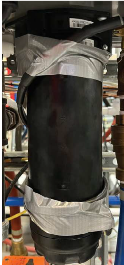
Figure 2 - Secure the bottom of the trace.
