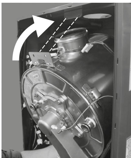
Figure 29 - Install heat exchanger to water heater
