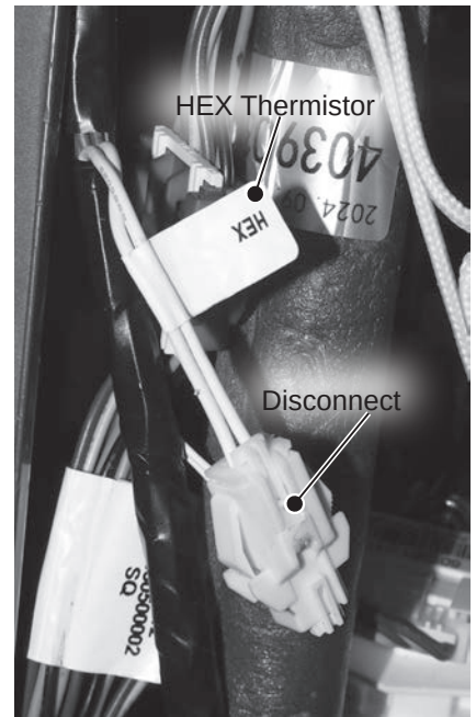
Figure 43 - Disconnecting HEX thermistor
