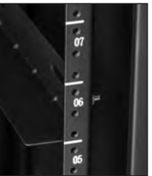
RACK U NUMBERS PRINTED ON RAILS
