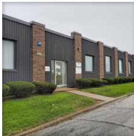
VIKING PUMP CANADA Windsor, Ontario, Kanada
