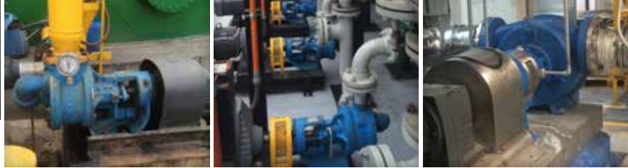
124A (icke-mantlad, packning) 224A (mantlad, packning) 324A (mantlad, packning)
