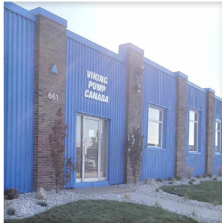
VIKING PUMP CANADA Windsor, Ontario, Canada
