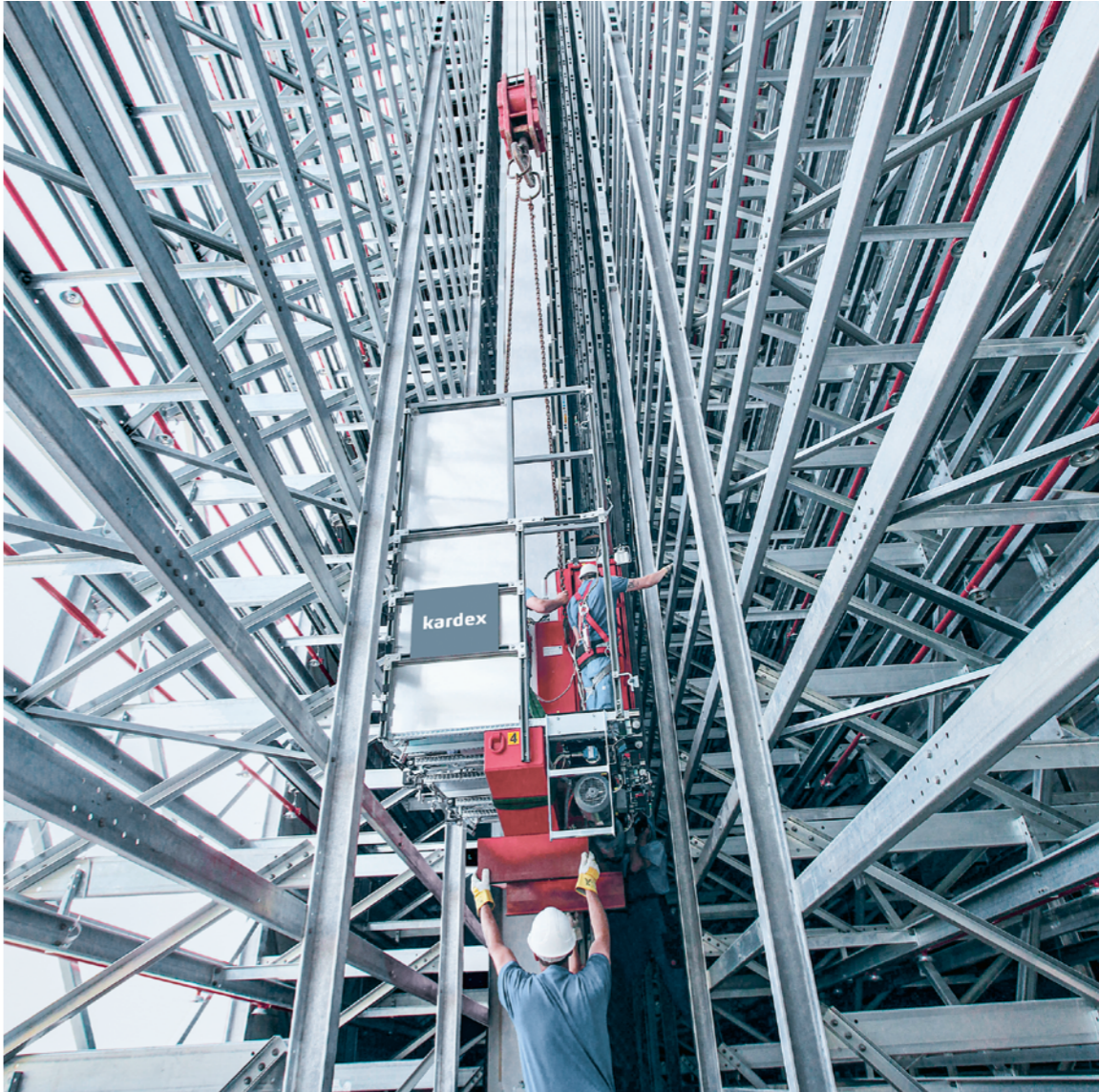
Construction of deep-freeze high-bay warehouse
