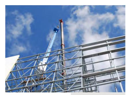
The storage and retrieval machines were installed via the roof.
