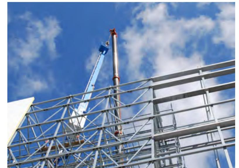
The storage and retrieval machines were installed via the roof.
