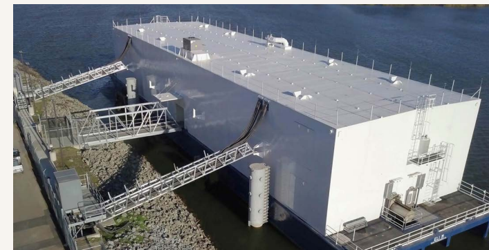
Nautilus Data Center
