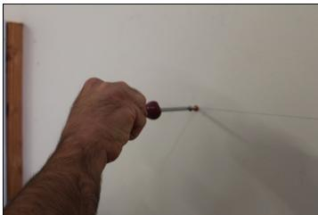
(8) Insert screws into anchors leaving 1/4" space.
