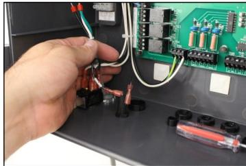
(17) Feed main power wires through conduit fitting.
