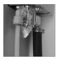
Route the tubing as shown and secure properly.
