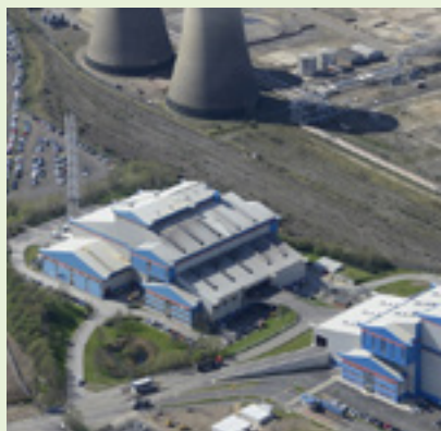
SUEZ's Haverton Hill energy-from-waste site
