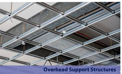
Used to build structural grids that support lighting, cable management, and mechanical components.
