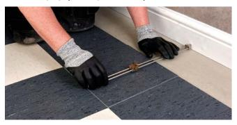
Figure 6 Measuring a tile using a scriber
