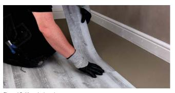
Figure 1 Setting planks out
