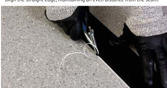
Figure 1 Grooving the seam
