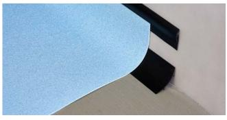
Figure 8 CS-N capping strips
