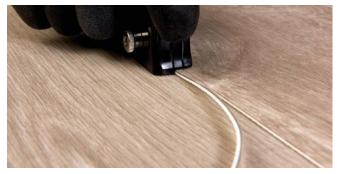
Figure 5 Cutting in the seams
