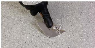
Figure 5a Final trim after the weld has cooled (Spatula Trimming Knife)
