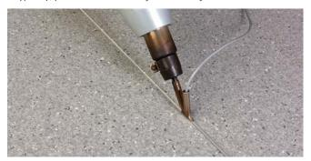
Figure 2 Applying the weld
