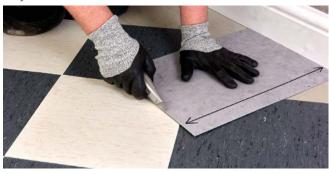
Figure 8 Cutting the perimeter tiles (diagonal cut)
