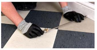
Figure 9 Cutting the tiles using a scriber (diagonal cut)
