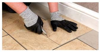
Figure 6 Measuring using an overlapping tile
