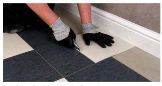
Figure 5 Measuring using an overlapping tile
