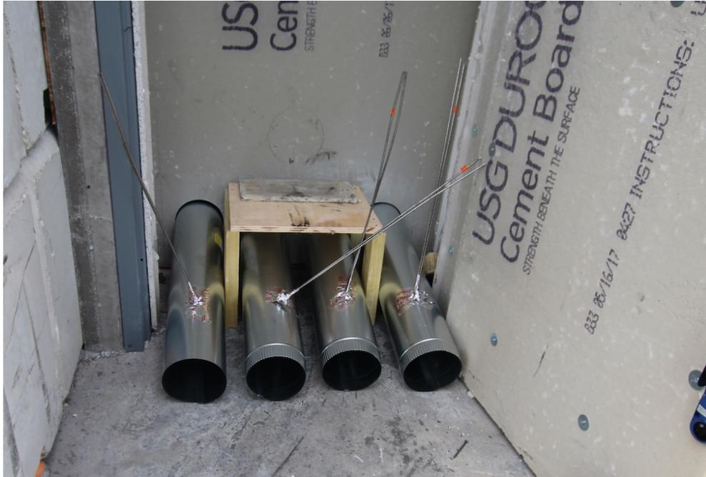
Figure 4.1: Leakage pipes (0.15 m (6 in.) diameter) installed in the side A wall of the basement.
