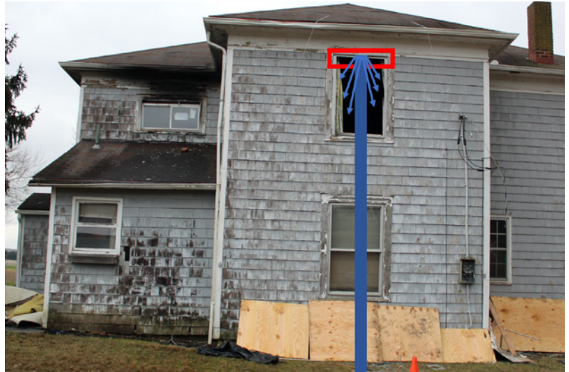
Figure 9. Example of improved water dispersion by leveraging exterior water directed off of a window frame.
