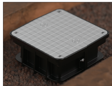
Gravel filled in, in 3"-6" (76 mm - 152 mm) increments, and then hand- or machine-tamped.
