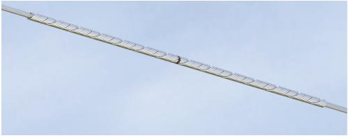
Repair Rods Installed on OPGW
