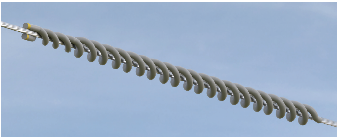
Subsented Spiral Vibration Dampers
