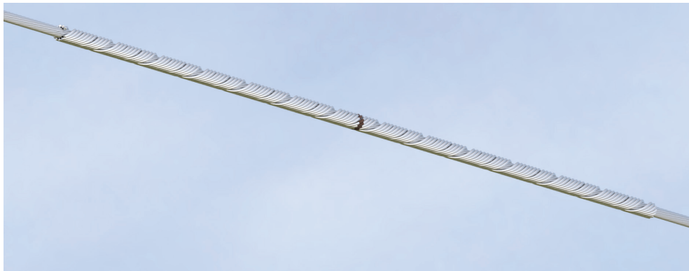
Repair Rods Installed on OPGW
