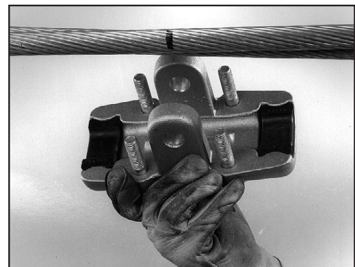
ALIGN BASE WITH MARK ON TWISTED PAIR CONDUCTOR
