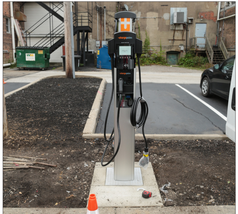
Completed foundation installation, with an attached charger.
