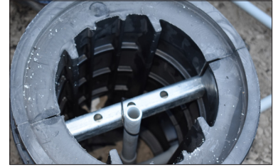
Conduit can be tie wrapped or wire tied to the middle bar for support.
