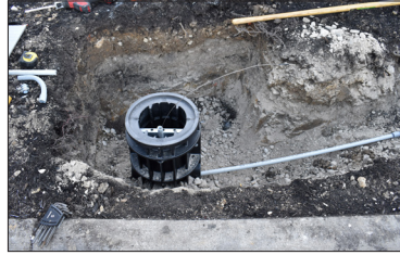
Ground prepared for installation of foundation; conduit ran and routed through open port to middle bar.
