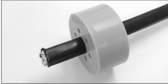
**Step #4** Remove the cable sheath per your accepted company practices. Leave 3" (76 mm) of the strength member to trim later.
