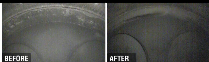
Combustion Chamber A
