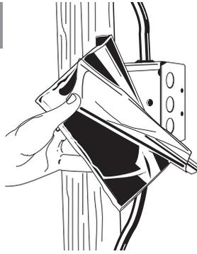
Align pad to the side of box partially overlapping the stud and adhere. Work to opposite side of the box to the edges.
