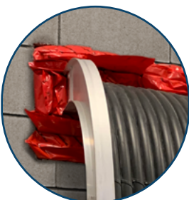
SpecSeal SSB Intumescent Firestop Pillows
