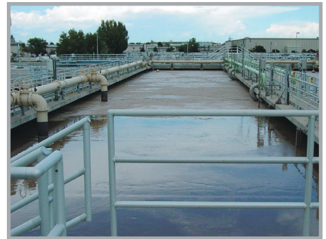
Award-winning Sand Creek Water Reuse Facility in Aurora, Colorado treats 5 MGD utilizing a Biological Nutrient Removal (BNR) system. Their effluent has ammonia less than 0.1 mg/L and phosphorous at 0.05 mg/L. (Photos courtesy of Sand Creek Water Reuse Facility.)
