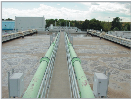
Award-winning Sand Creek Water Reuse Facility in Aurora, Colorado treats 5 MGD utilizing a Biological Nutrient Removal (BNR) system. Their effluent has ammonia less than 0.1 mg/L and phosphorous at 0.05 mg/L. (Photos courtesy of Sand Creek Water Reuse Facility.)
