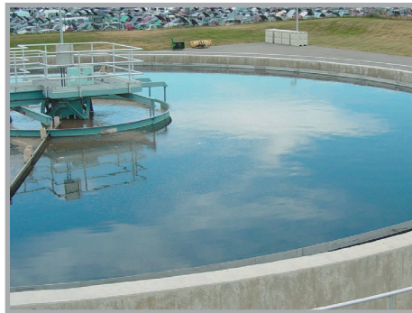
Award-winning Sand Creek Water Reuse Facility in Aurora, Colorado treats 5 MGD utilizing a Biological Nutrient Removal (BNR) system. Their effluent has ammonia less than 0.1 mg/L and phosphorous at 0.05 mg/L. (Photos courtesy of Sand Creek Water Reuse Facility.)
