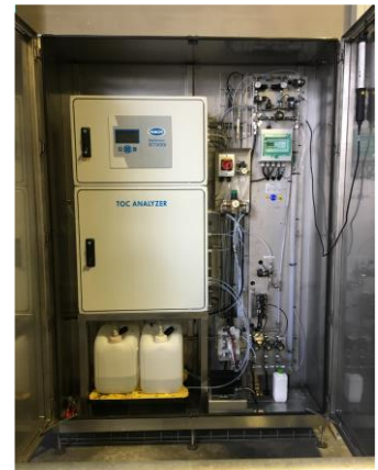
Hach BioTector B7000i Dairy with Venturi Vacuum Sampler at MEGGLE in Wasserburg
