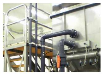
suspended solids levels in DAF influent and use these ongoing readings to automatically control chemical feed dosage. The signal from the sensor is linked to the plant's DCS or SCADA system using a full-scale 4-20 mA
