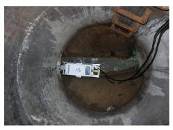
DDS Flo-Dar Sensor installed in a manhole
