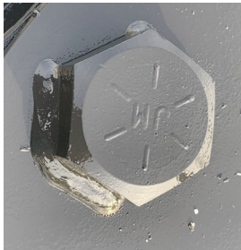
FIGURE 3.7A BOLT HEAD BEAD WELD & ASSEMBLY
