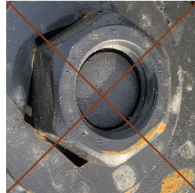
FIGURE 3.7B BOLT THRU NUT
