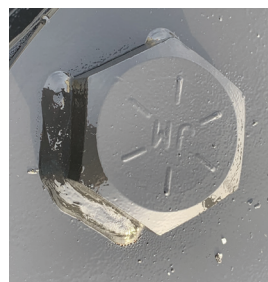
FIGURE 3.7A BOLT HEAD BEAD WELD & ASSEMBLY
