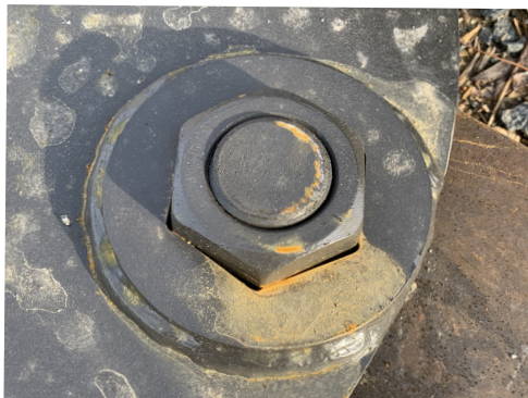
Figure A2 Bolt Thru Nut
