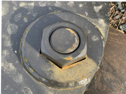
Figure A2 Bolt Thru Nut
