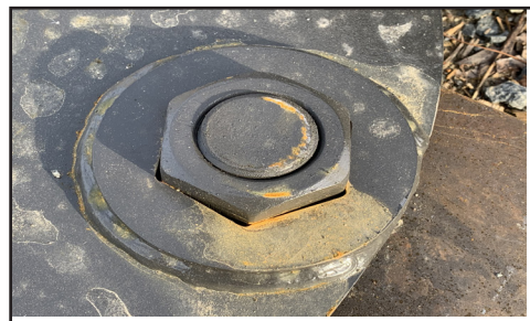
Figure 4.7b Bolt Thru Nut
