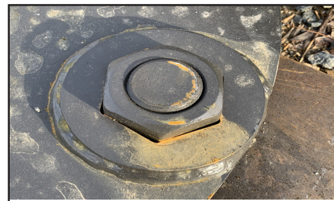
Figure 4.7b Bolt Thru Nut
