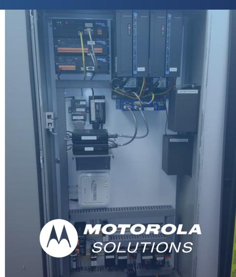
The ACE3600 RTU excels in SCADA environments, offering unmatched flexibility and robustness for complex data management and secure communications in critical infrastructure operations.
