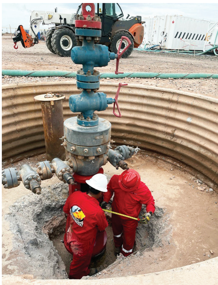
FIG. 1. Well control specialists conduct a wellhead audit to assess the integrity and equipment condition in a mature oil and gas infrastructure.
