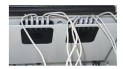
Insert the device cables into the cable management bracket.
